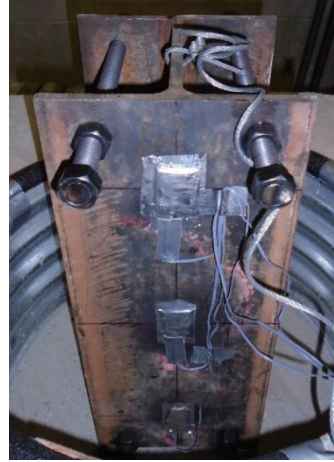
Figure 65. H pile instrumentation
