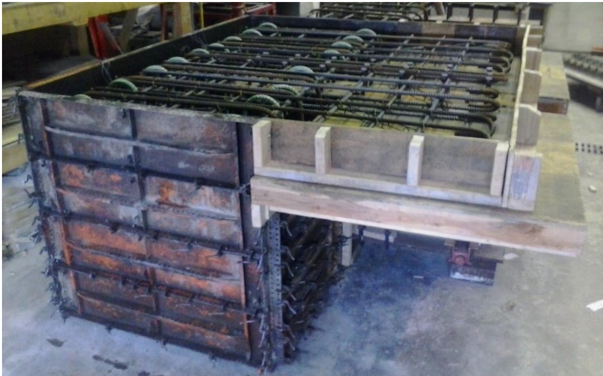
Figure 28. Integral diaphragm and deck, formwork and rebar
