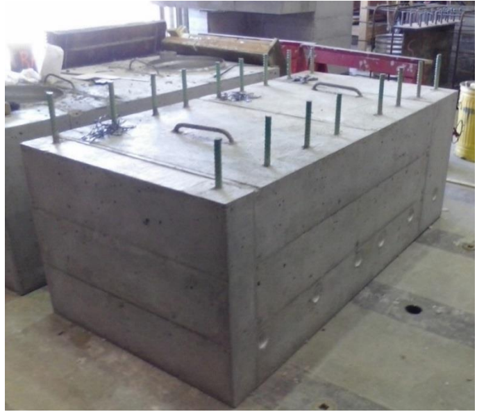
Figure 24. Grouted coupler pile cap
