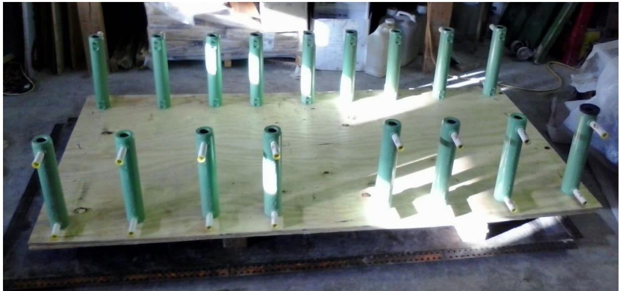
Figure 25. Grouted coupler template
