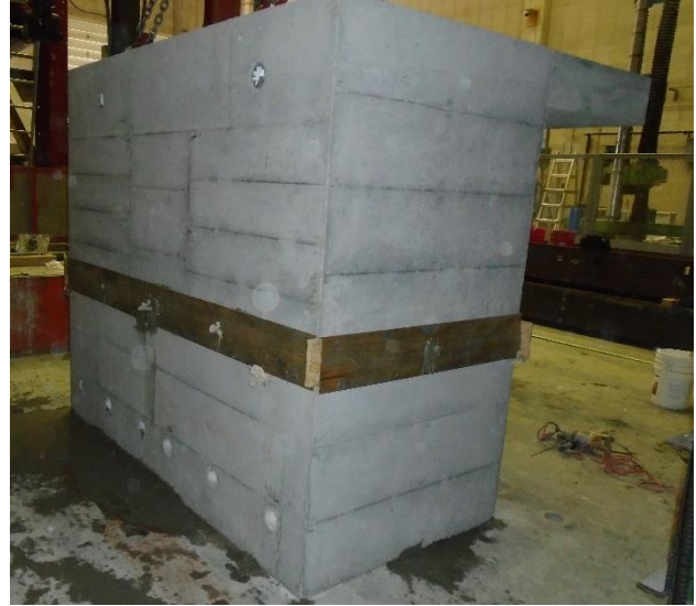
Figure 50. Grout bed formwork front
