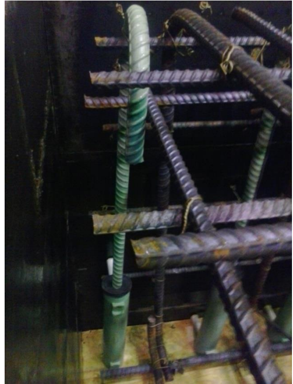
Figure 27. Grouted coupler and rebar
