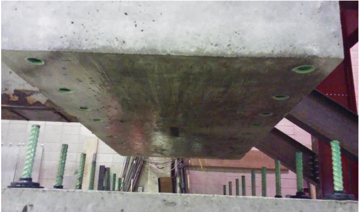
Figure 32. Integral diaphragm placement
