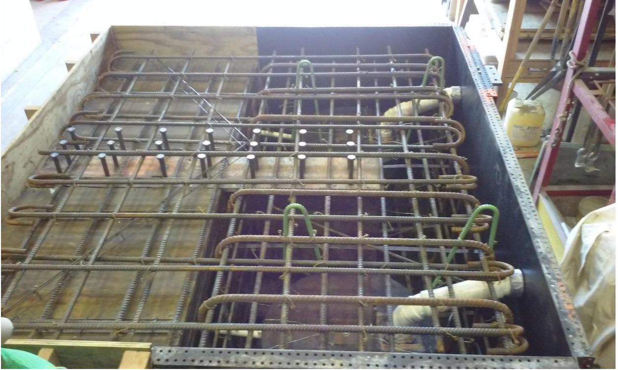
Figure 45. Integral diaphragm deck rebar
