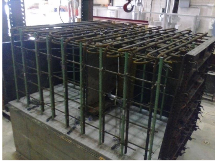
Figure 21. CIP integral diaphragm
