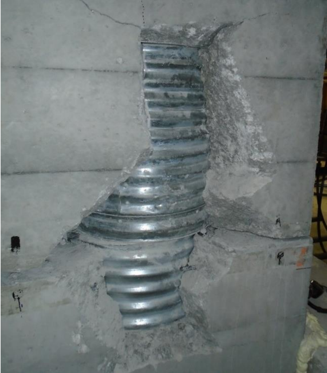
Figure 79. Pile coupler deconstruction
