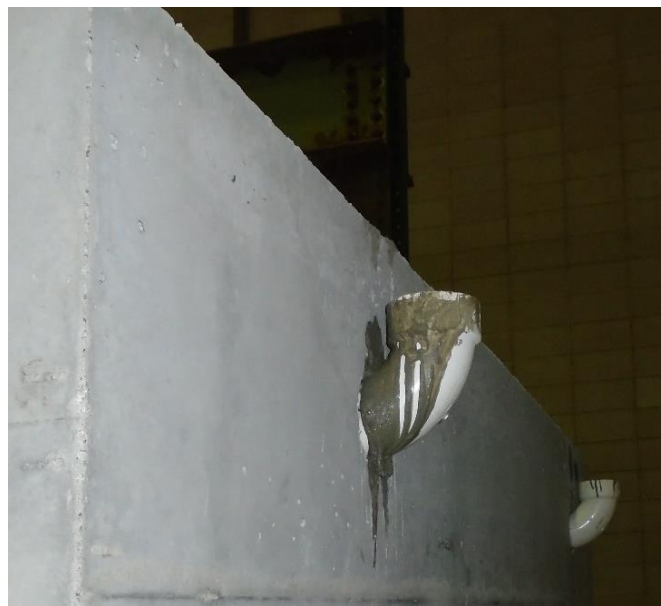
Figure 52. PVC pipe for receiving grout
