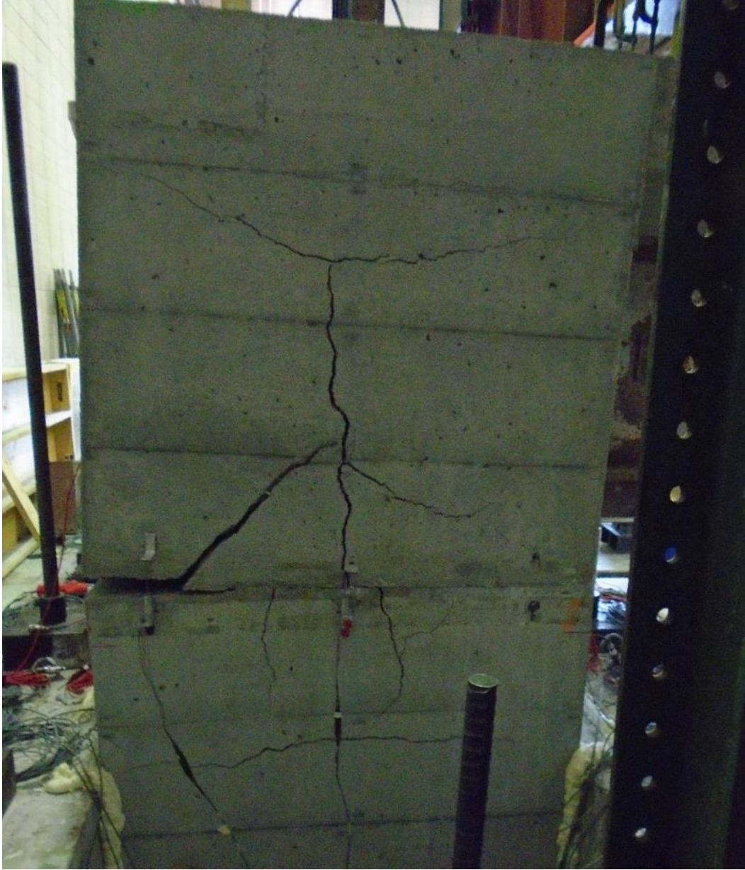
Figure 78. Pile coupler damaged East side
