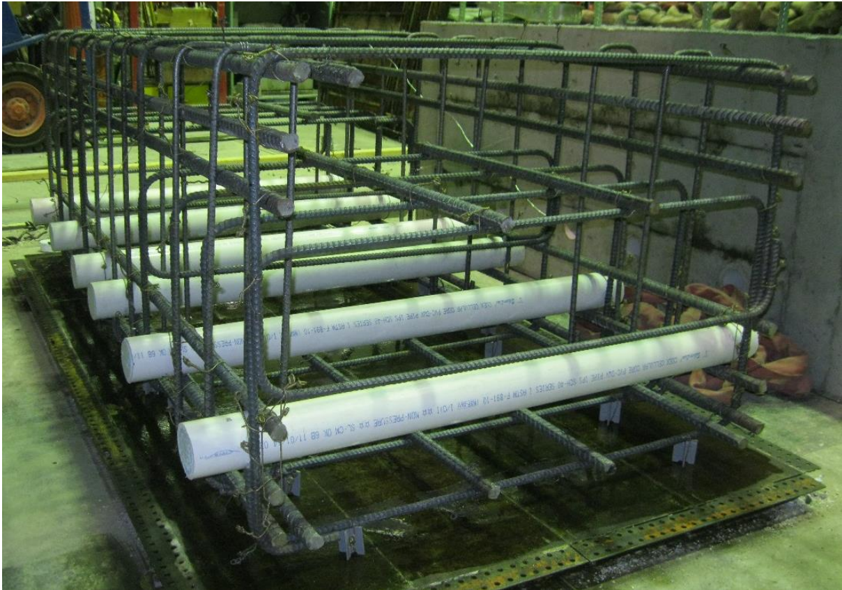
Figure 37. Pile cap rebar cage
