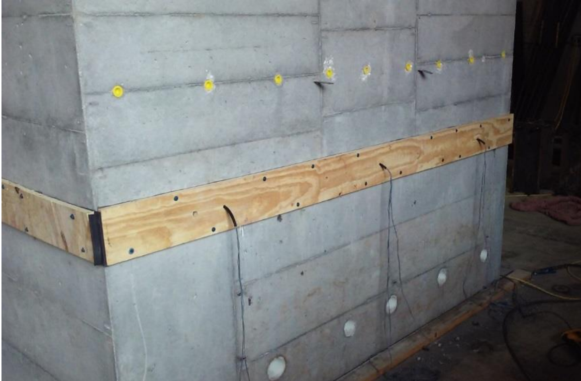
Figure 33. Grout bed formwork
