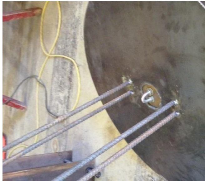
Figure 40. CMP lid with rebar guides and U-bolt
