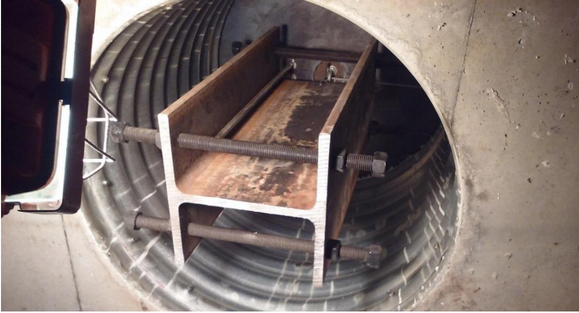
Figure 47. Suspended HP sections
