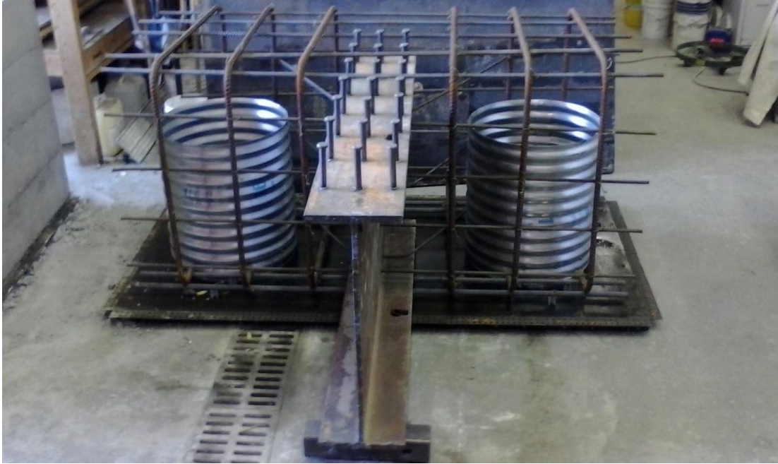
Figure 43. Integral diaphragm rebar cage
